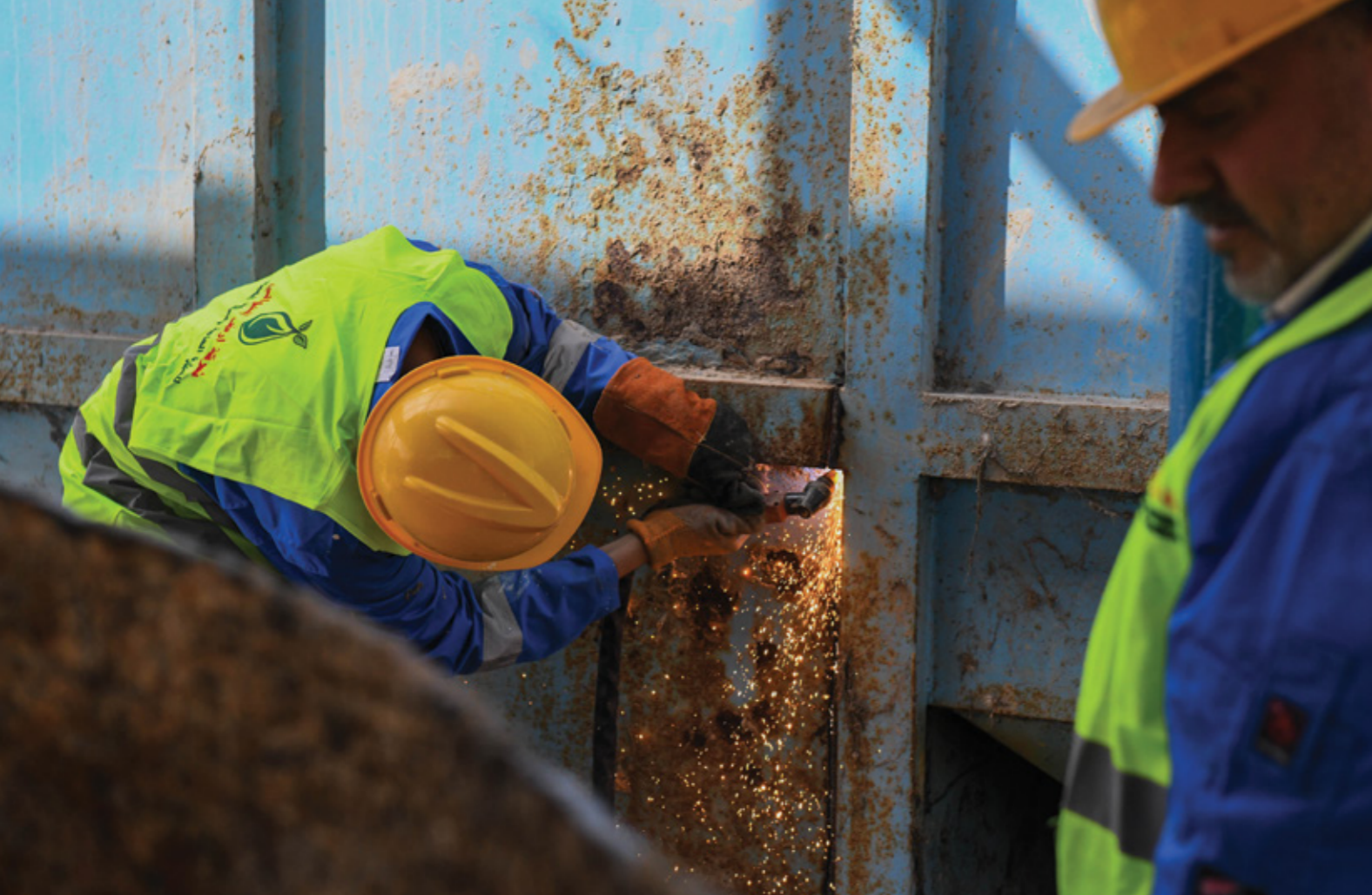
A water desalination unit in Thi-Qar is being rehabilitated to improve access to safe water under UNDP Iraq's Human and Biodiversity Resilience in the Mesopotamian Marshes Project, funded by the Government of Canada. © UNDP Iraq / Mahdi Al-Saadawi
